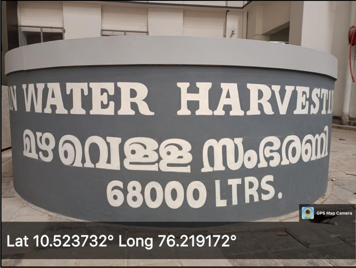
Rain Water Harvesting at Academic(Science) Block
