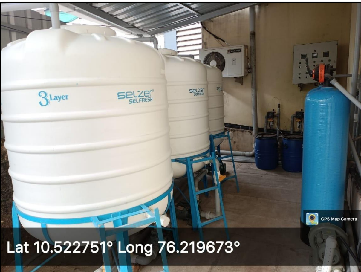
Waste Water Recycling Plant in Administrative Block
