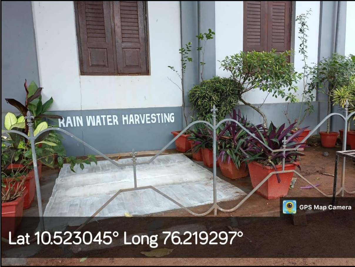
Rain Water Harvesting at Administrative Block
