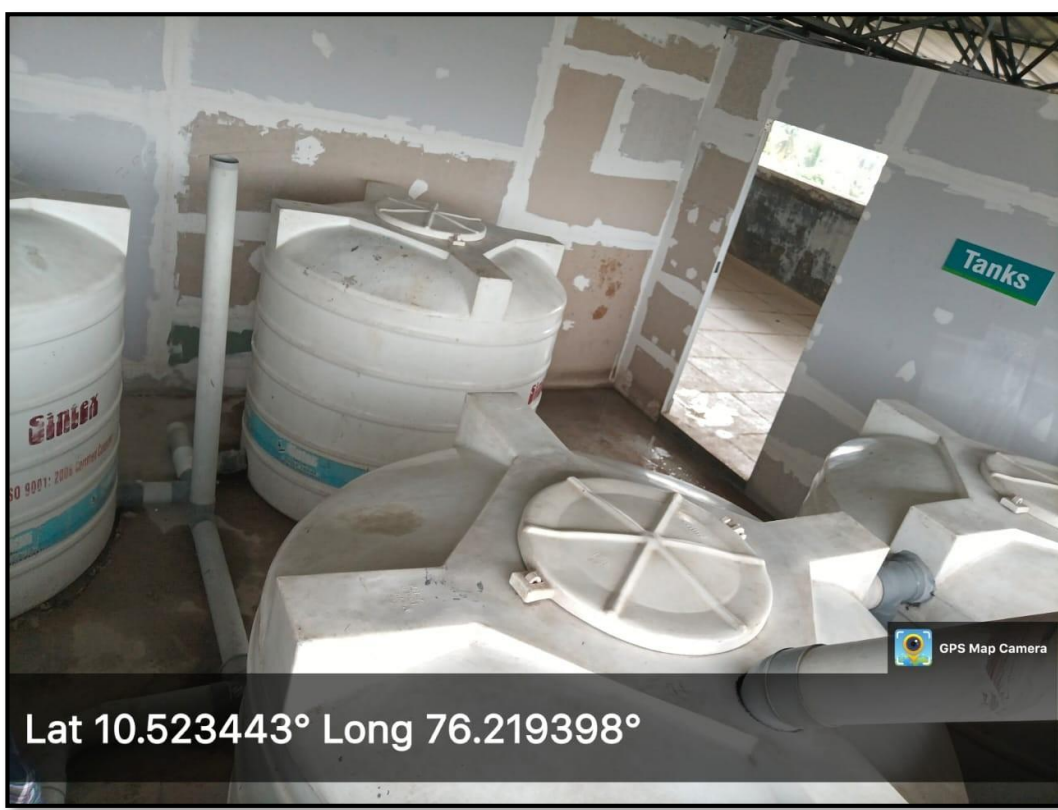
Rain Water Collecting Tanks at Academic Block
