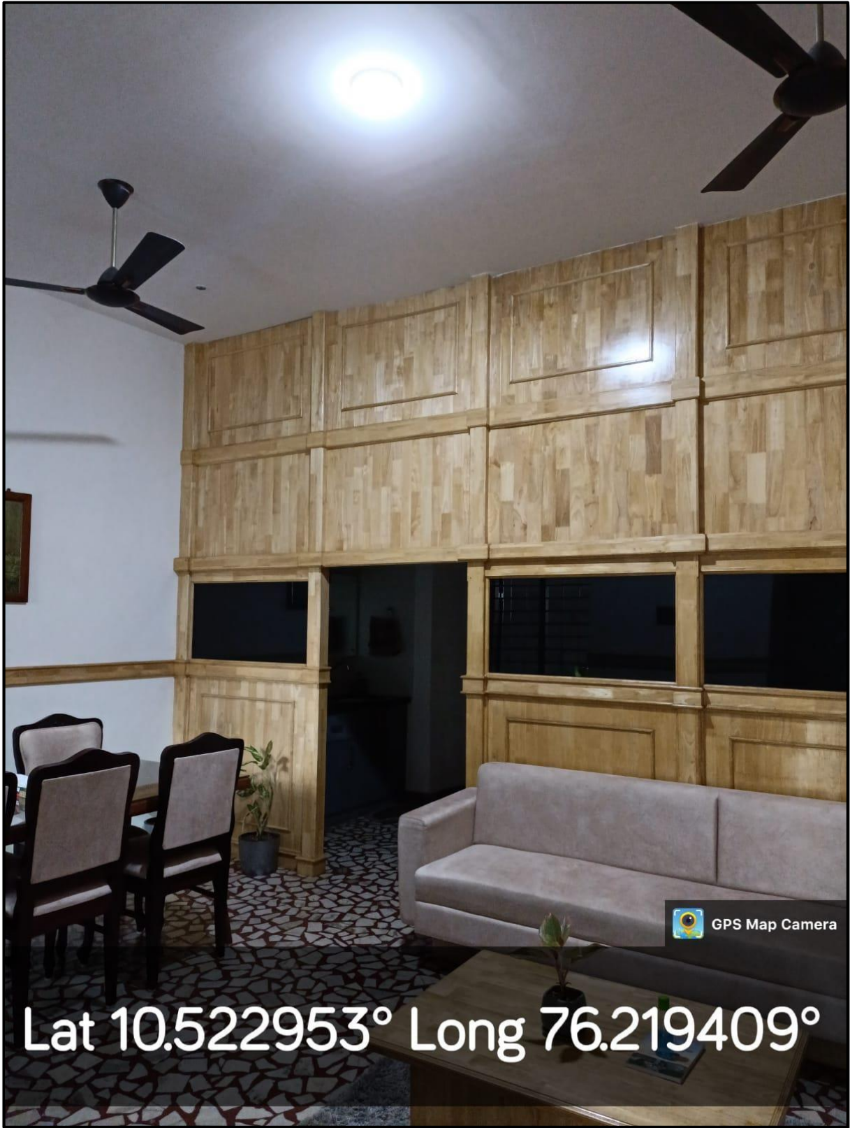
Sensor Light in Administrative Block Guest Room
