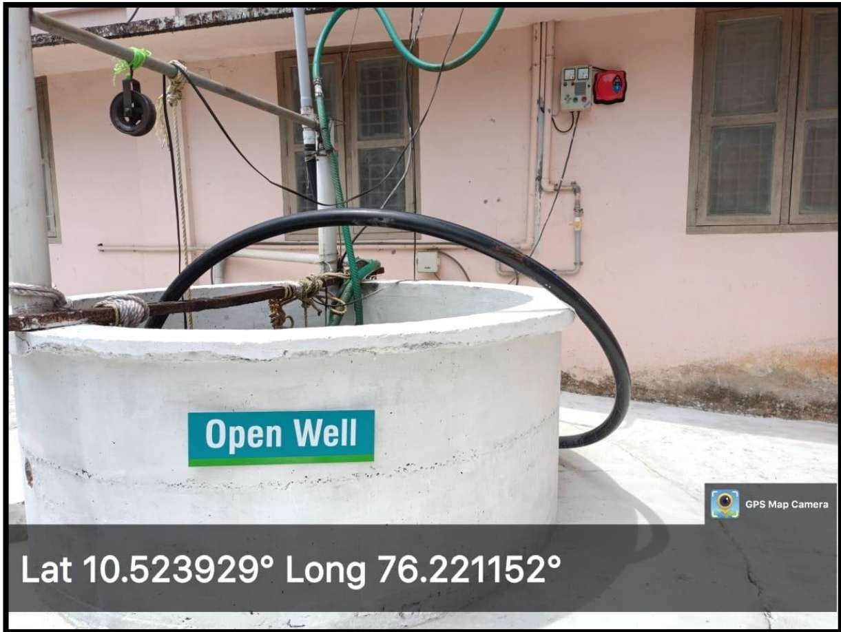
Open Well Recharging in the Jubilee Block
