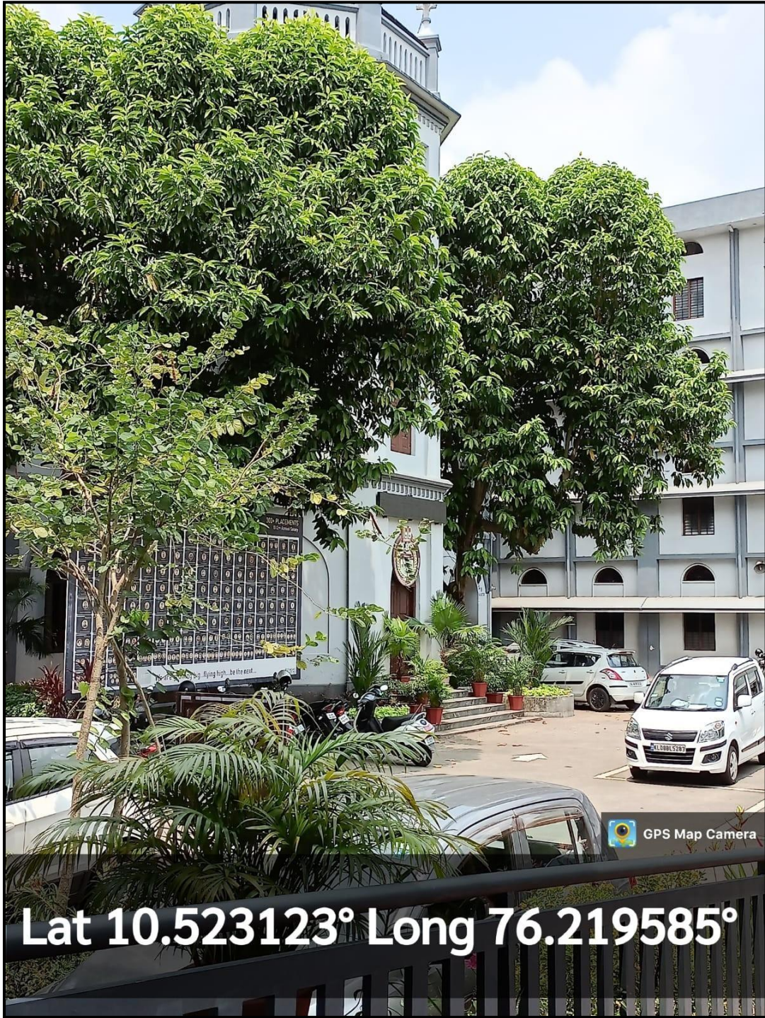
Landscaping in Administrative(Main)Block
