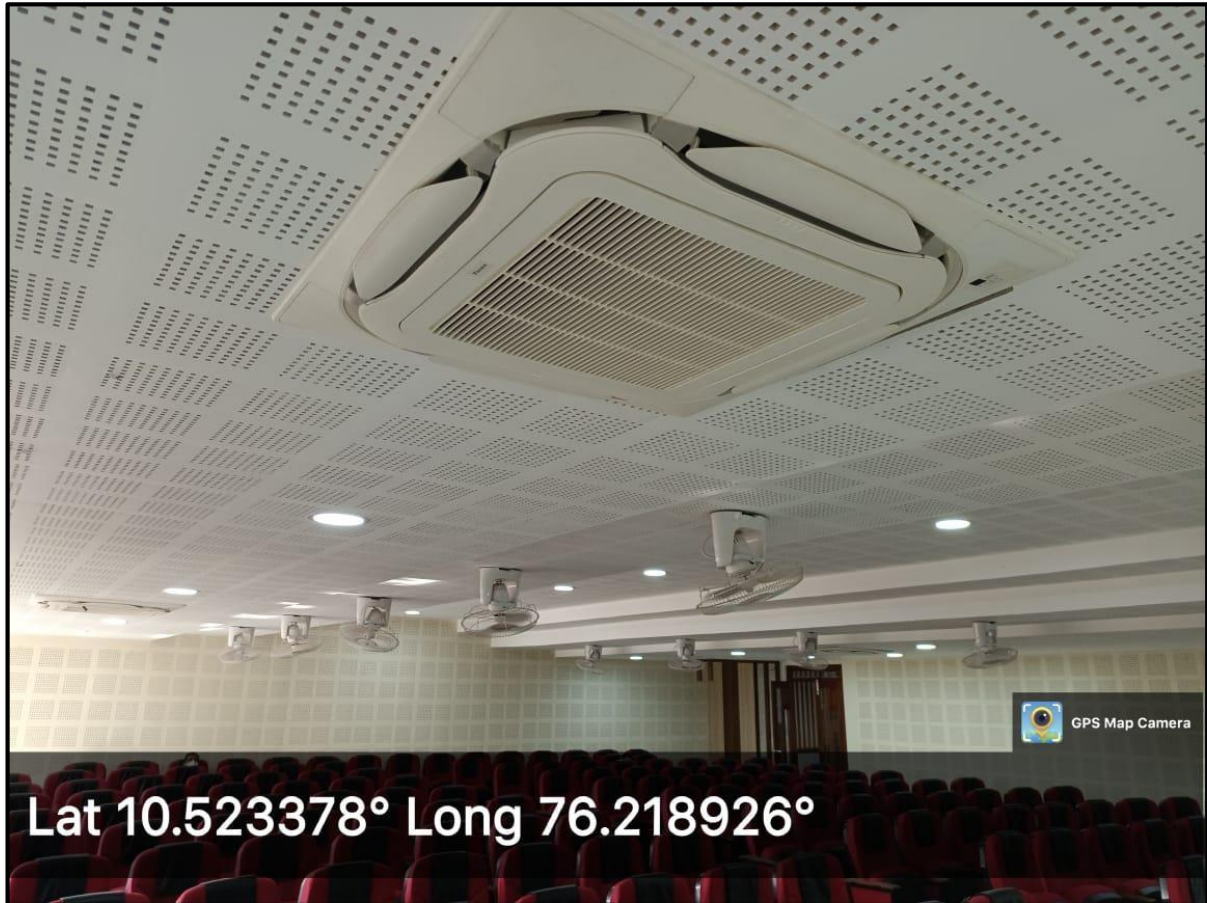
Daikin VRV IDU High Wall at Research Seminar Hall
