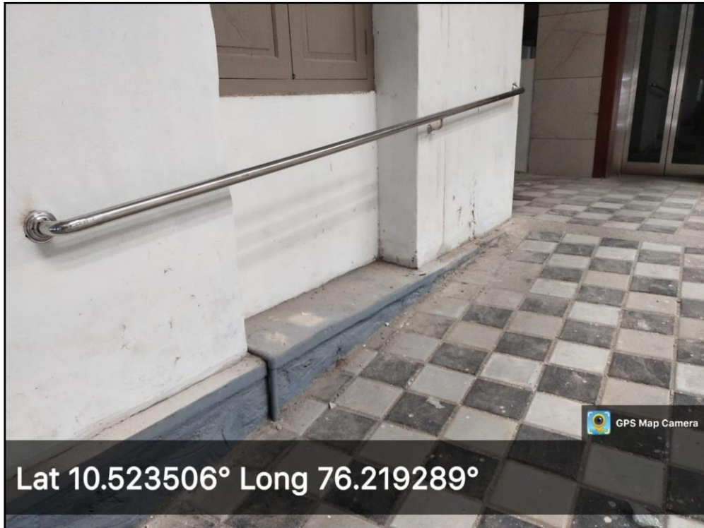
Ramp near to the lift in Academic block
